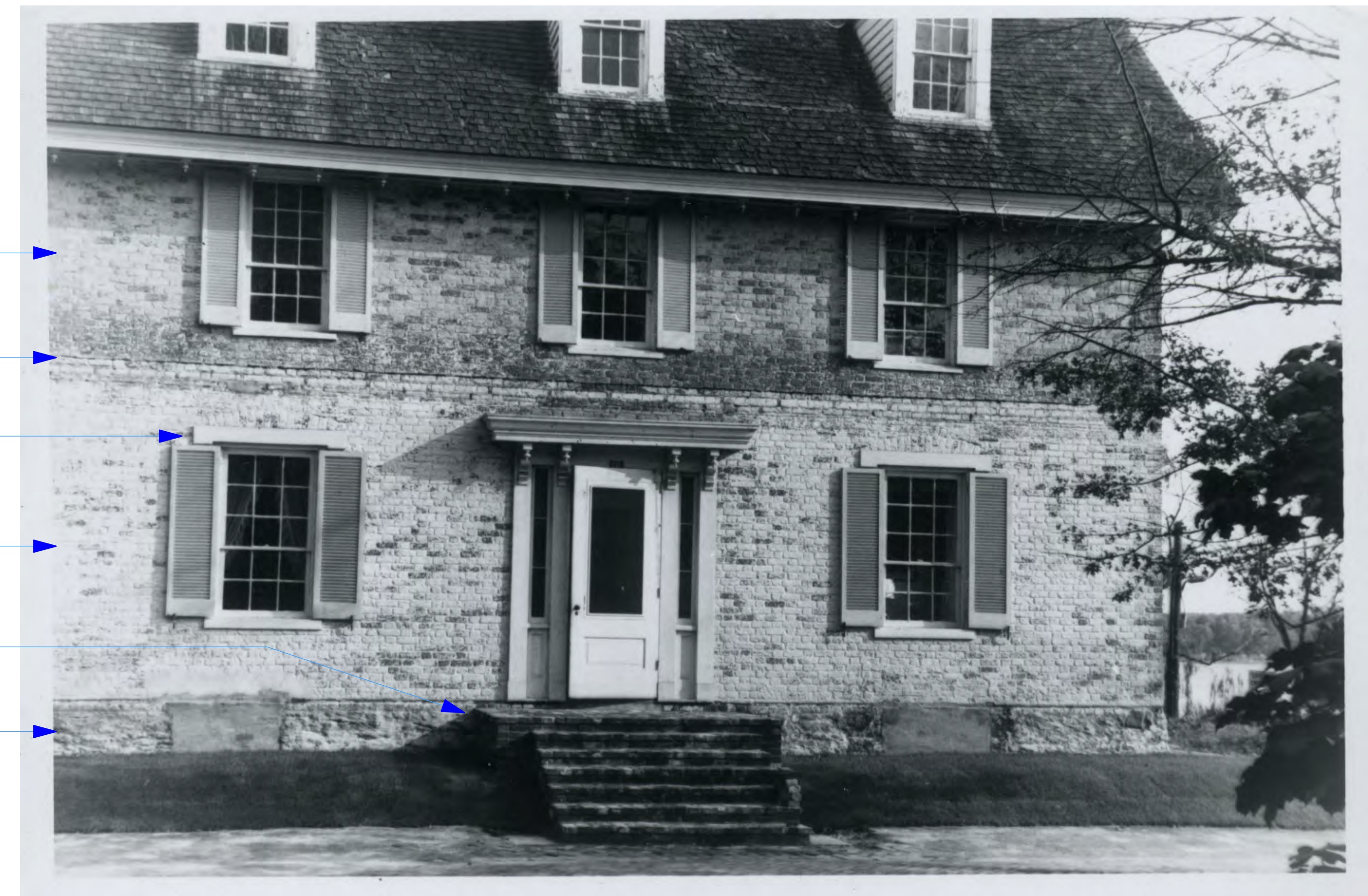
WATER ST VIEW DURING CONSTRUCTION - Ca 1974
