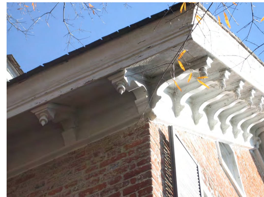
1860s CORNICE FROM SW
