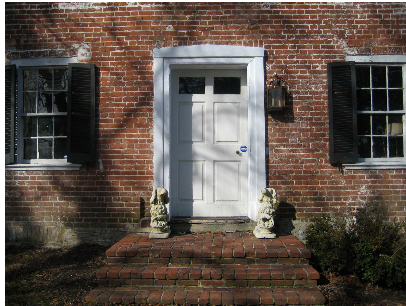
RIVERFRONT ENTRY 'AS IS' AN 1860s ITALIANATE ARCHITRAVE ON AN 18TH CENTURY ADDITION WITH A 1974 "GEORGIAN" STOOP
