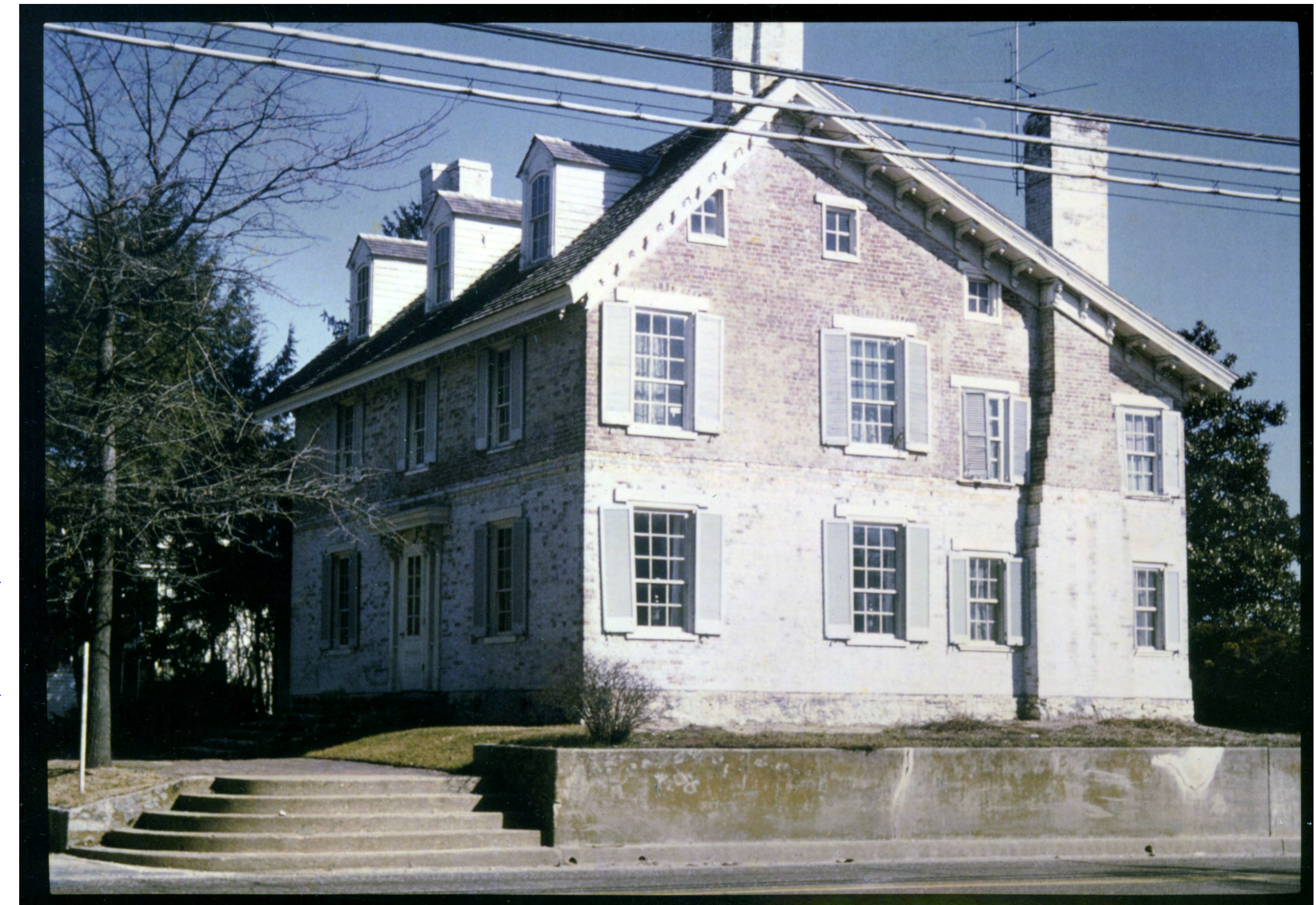
FROM SW DURING CONSTRUCTION - Ca 1973
