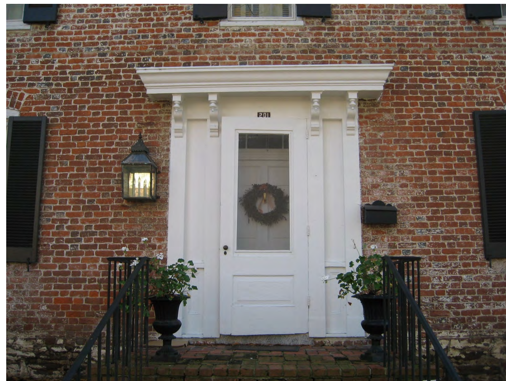
WATER STREET ENTRY 'AS IS' AN 1860s ITALIANATE ARCHITRAVE ON A 1760s GEORGIAN HOUSE WITH A 1974 "GEORGIAN" STOOP
