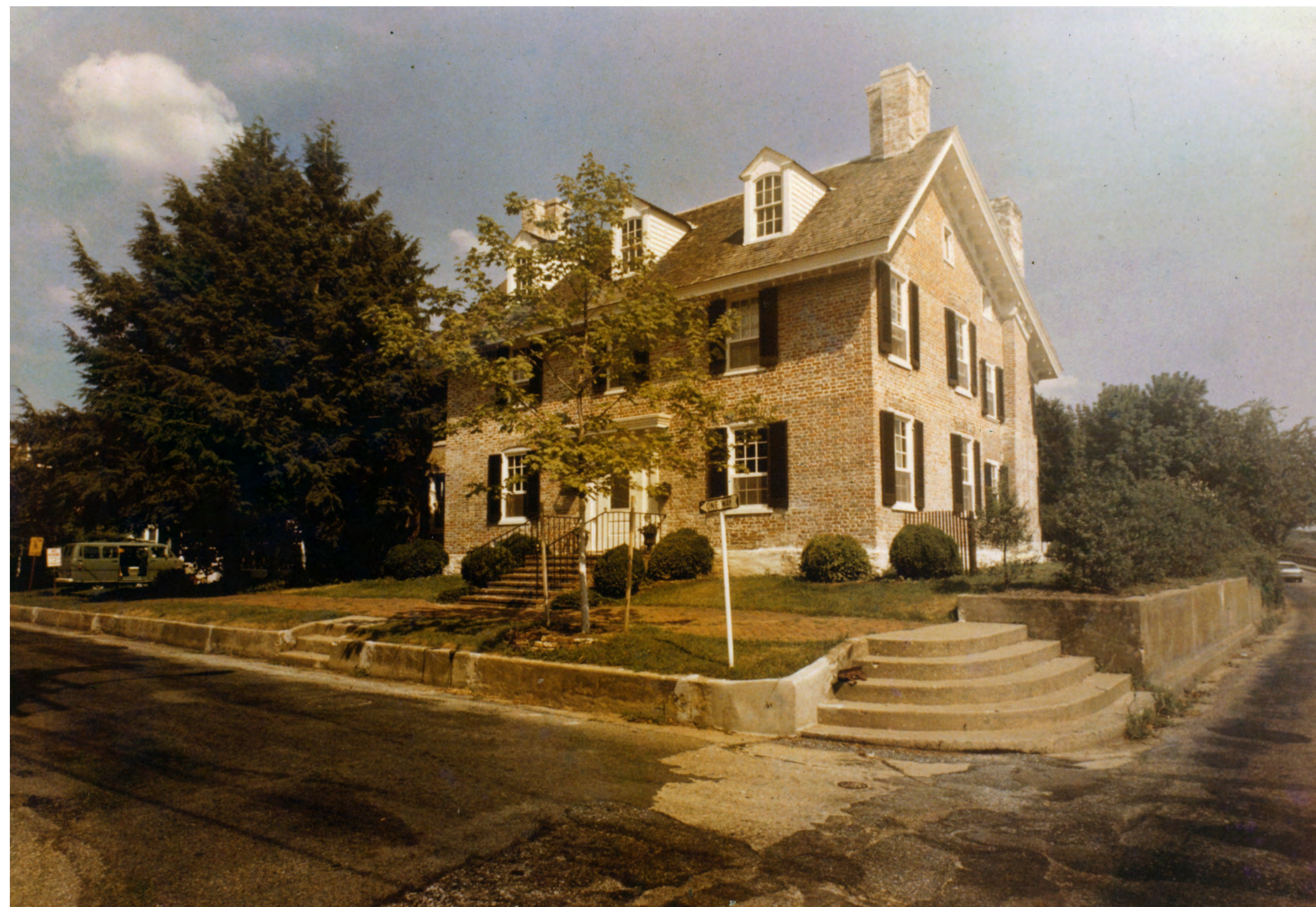
VIEW FROM INTERSECTION - DEC 1974
