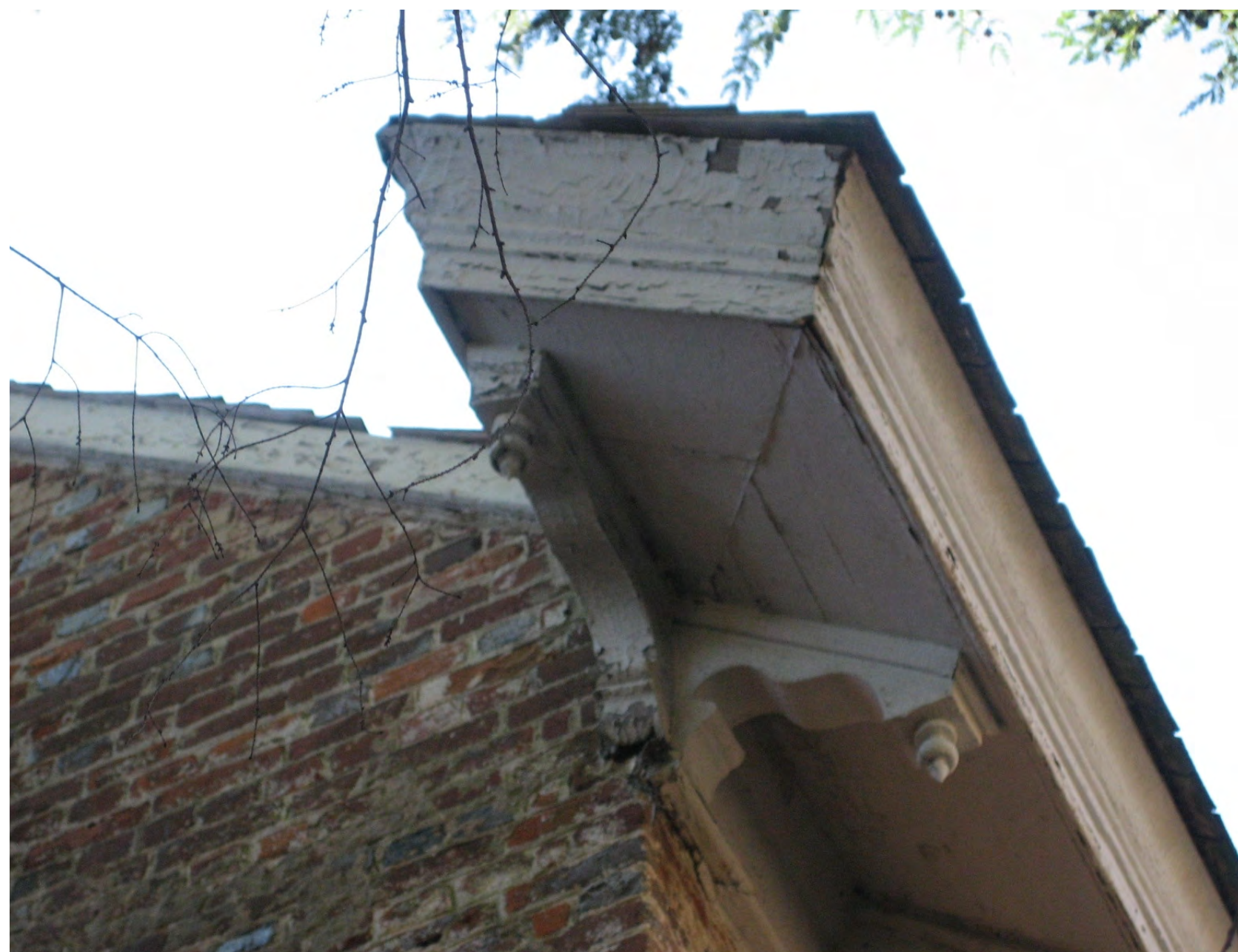
1860s CORNICE FROM WATER ST AN 1860s ITALIANATE CORNICE ON A 1760s GEORGIAN HOUSE THE ORIGINAL 1760s VERGEBOARD?
