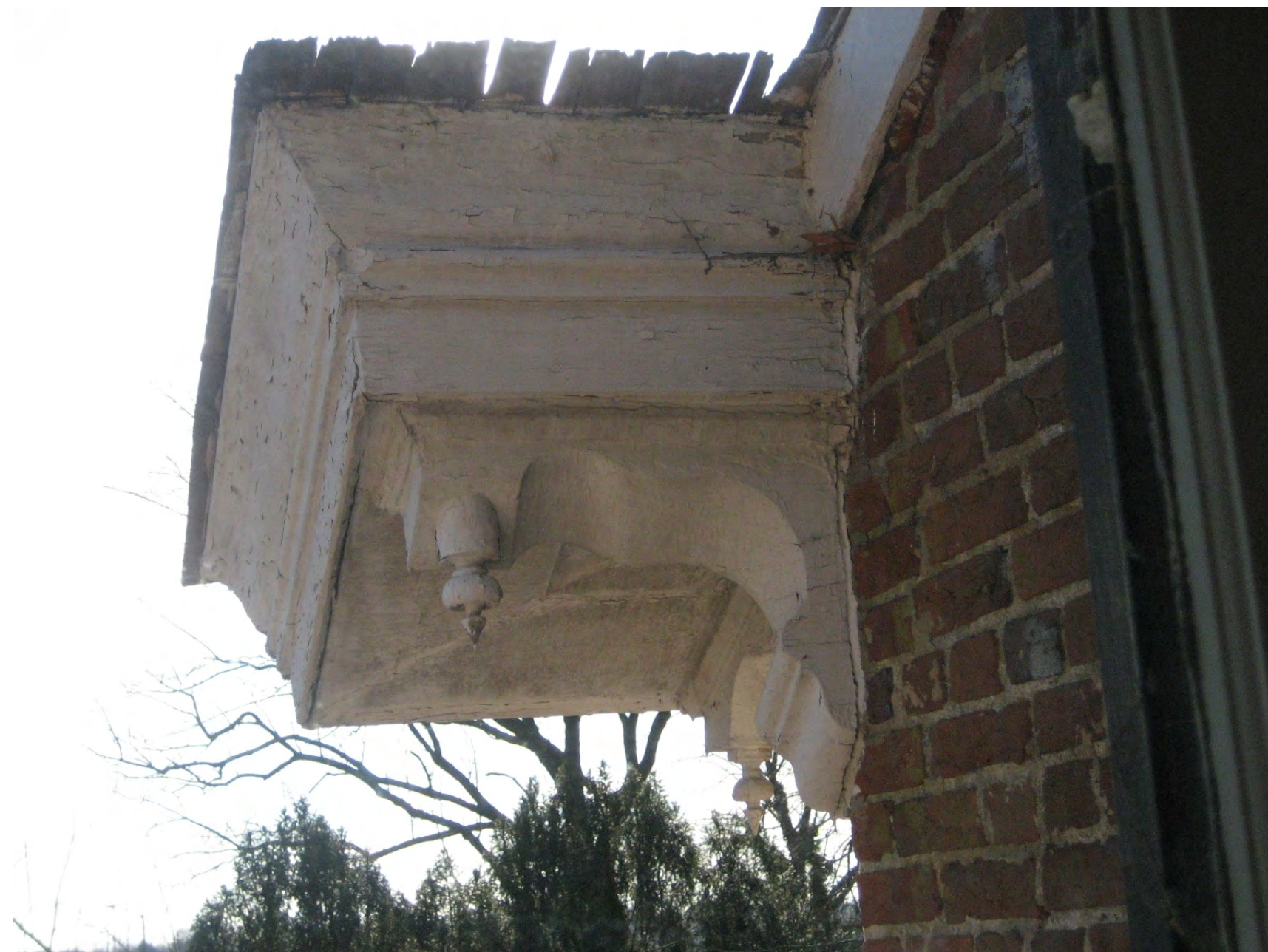
EAVE EXTENSION AT 1770s RIVERSIDE WALL AN 1860s ITALIANATE CORNICE, ON A 1770s ADDITION (AS SEEN FROM THE 1860s BEDROOM).
